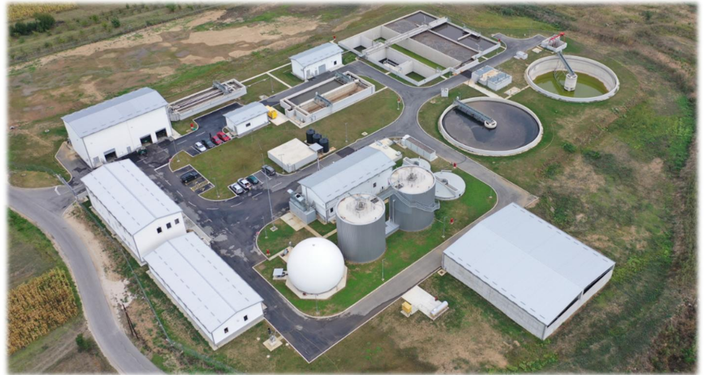
Aerial view WWTP Vranje (08.2022)
