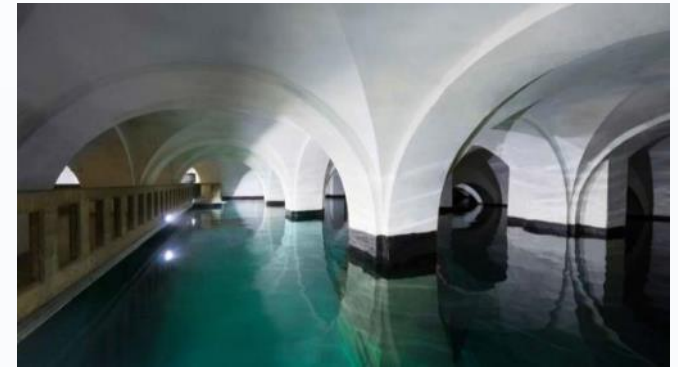
Water reservoir Rosenhügel (© Vienna Water, Novotny)
