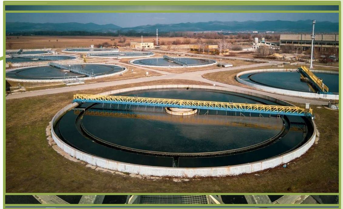
Secondary settling tanks 10 ps.
