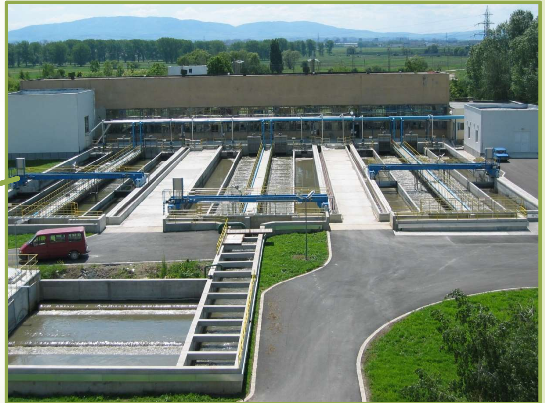
Sand and grease removal
