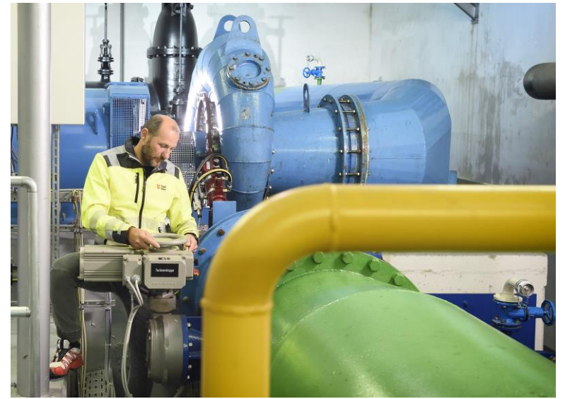
Water power plant
