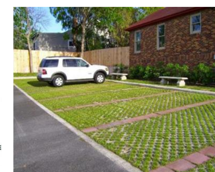
Fig.2 Greenery and filter strips at streets and general public space - Greenery besides public streets and permeable pavements & parking lots can be used to hold back stormwater or infiltrate it into the ground. Furthermore, cleaning is done by the natural layer and the plants contribute to the climate, clean air etc.
