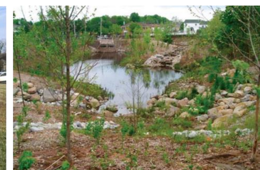
Fig3. Soil Retention basins/ Constructed wetlands for stormwater treatment- these are nature- based solutions for retention and primary cleaning of stormwater runoff (as well as emergency overflow of mixed systems).
