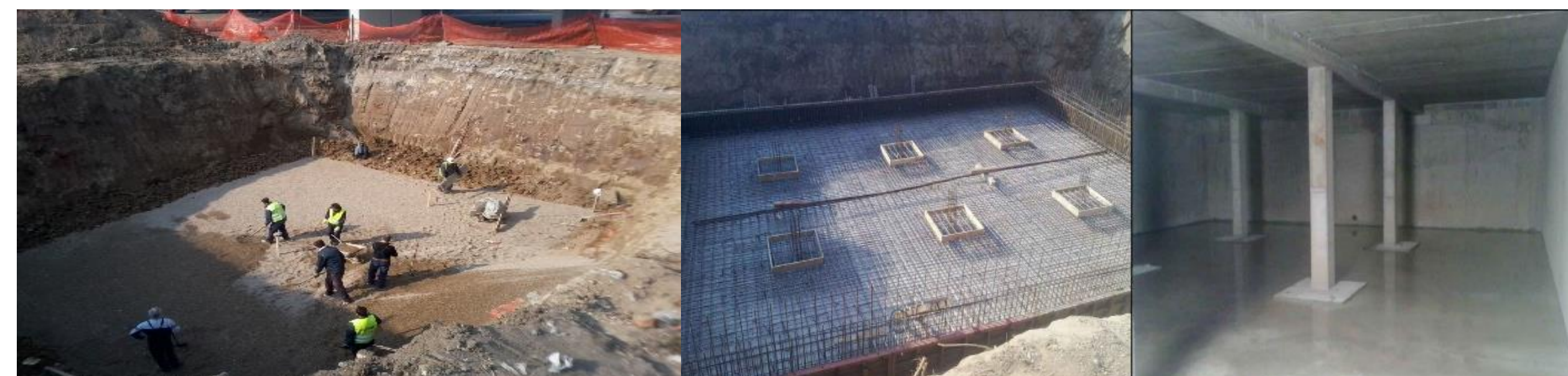
Figure 2. Retention in the construction phase
