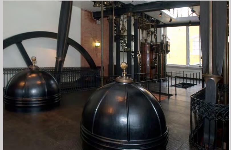
Ancient pumping station, Museu da Água, EPAL, Lisbon Photo: Américo Simas
