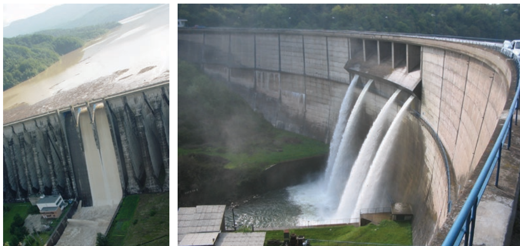
PHOTOGRAPH 3.4. View of Dams for Flood Protection
