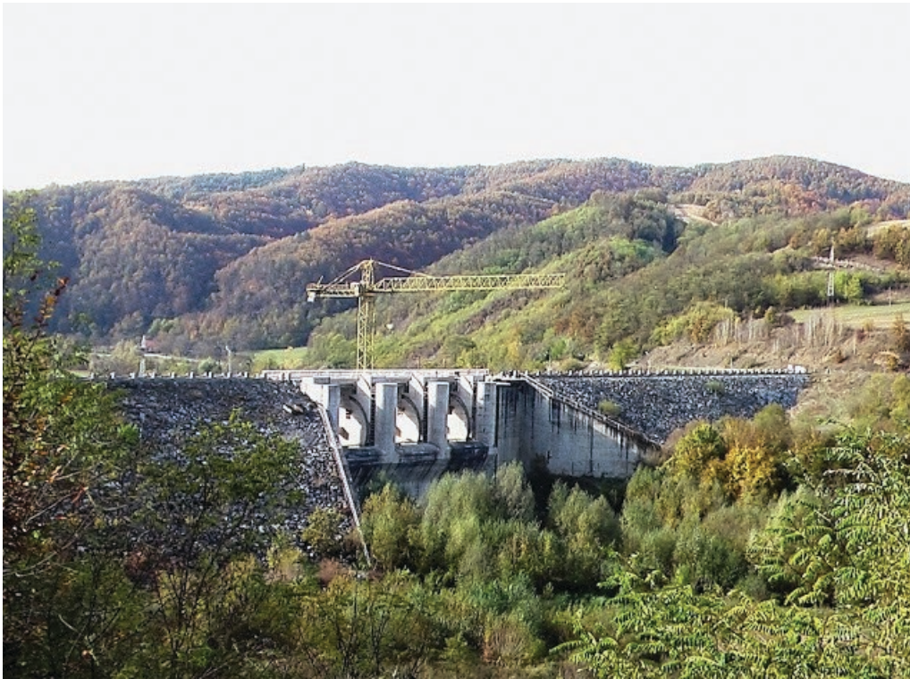
PHOTOGRAPH 3.9. View of the Mihăileni Dam
