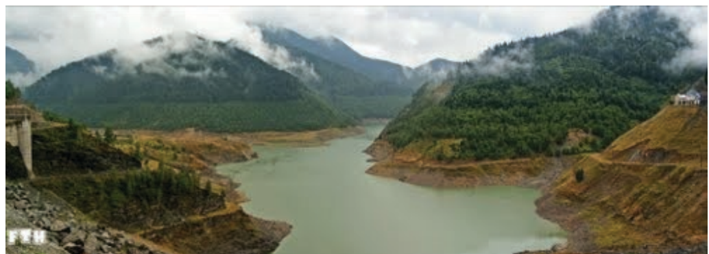
PHOTOGRAPH 3.10. View of the Gura Apelor Dam
