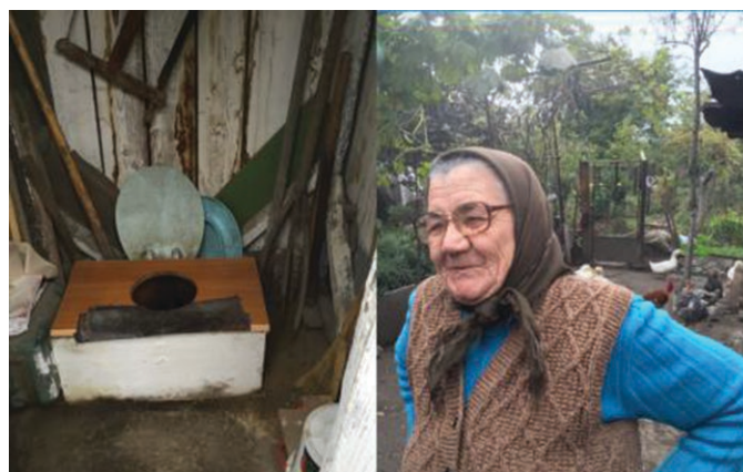
PHOTOGRAPH 2.2. Pit Latrine in Rural Romania
