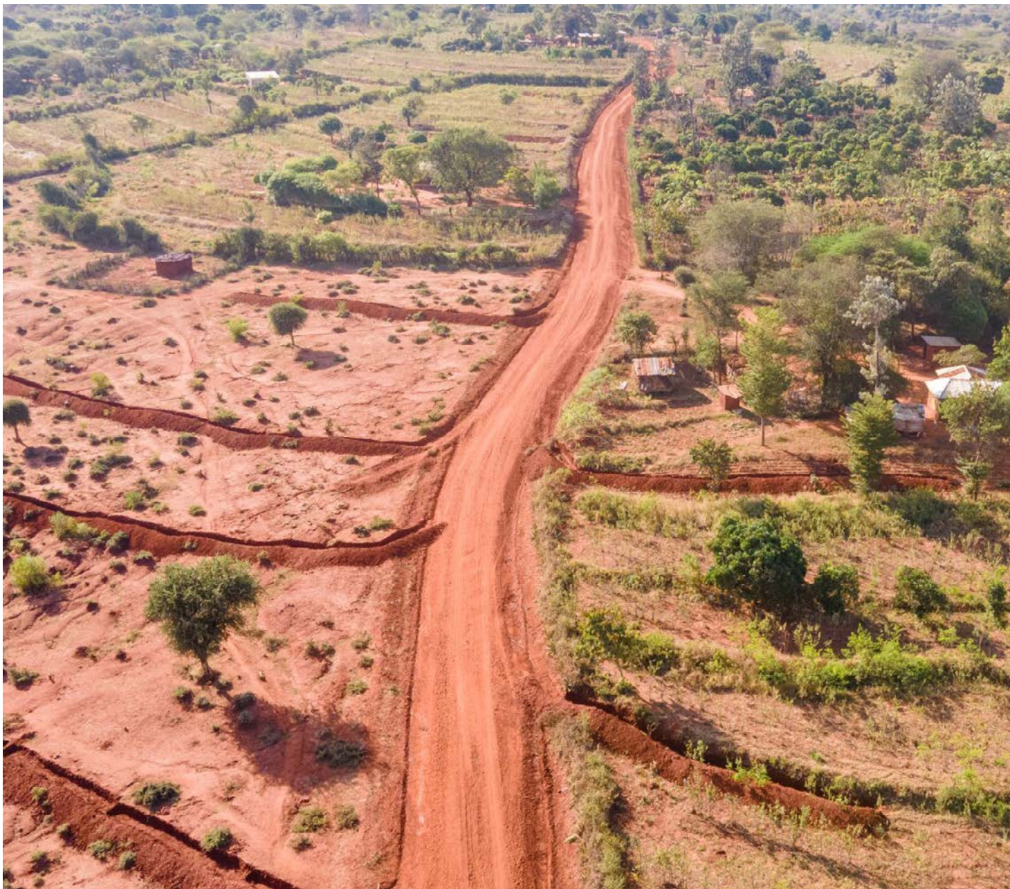
NBS, including run-off harvesting measures, installed along three kilometers of road for the "Drain to Gain Project", Kenya. Photo by MetaMeta.
