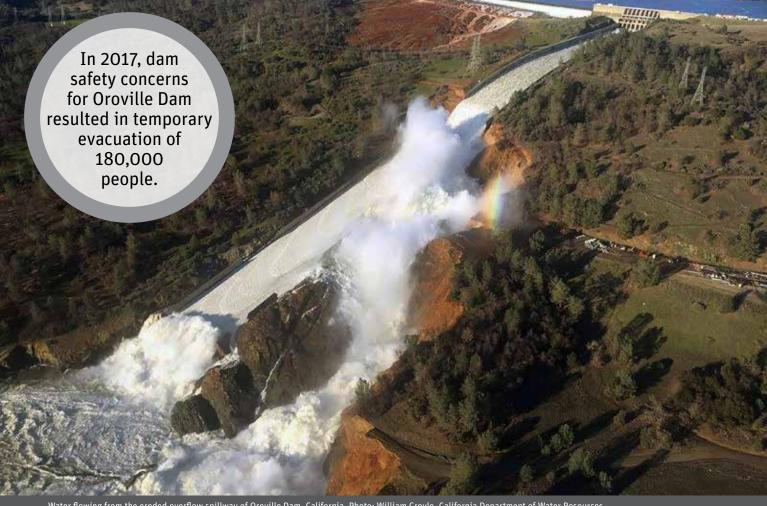
Water flowing from the eroded overflow spillway of Oroville Dam, California. Photo: William Croyle, California Department of Water Resources
