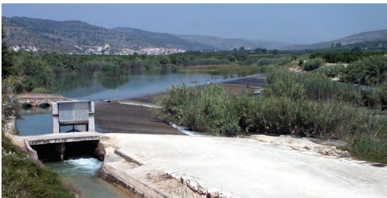
Image 3.2 Diversion weir of Carcaixent on the river Júcar, Spain
