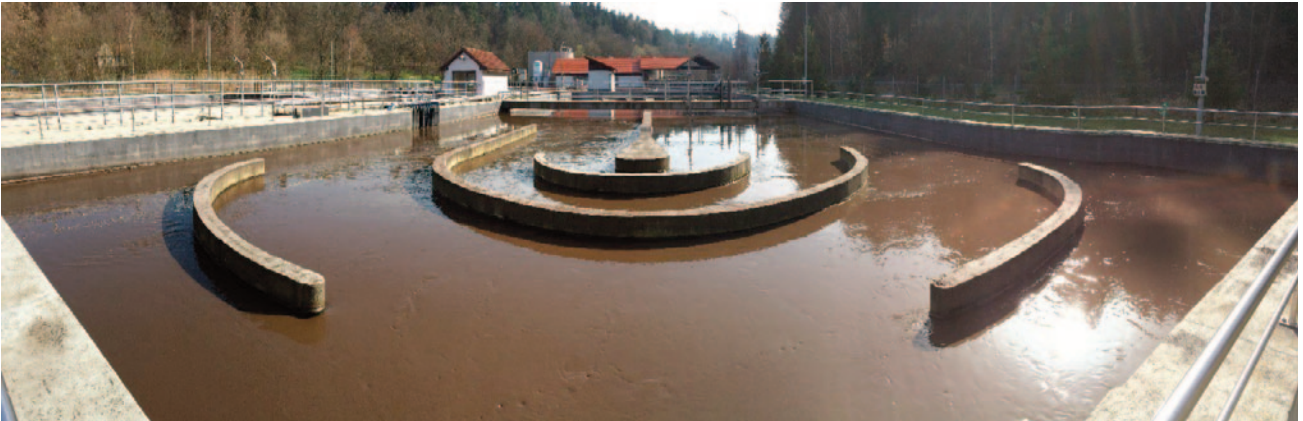
Wastewater treatment plant of Moravska Trebova modernised with the support of EU funds
