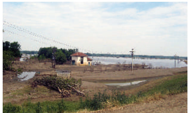
Water supply source of Obrenovac (Vic Bara) was flooded
