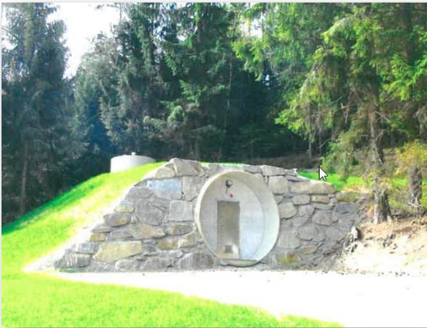
Cistern / space for technology
