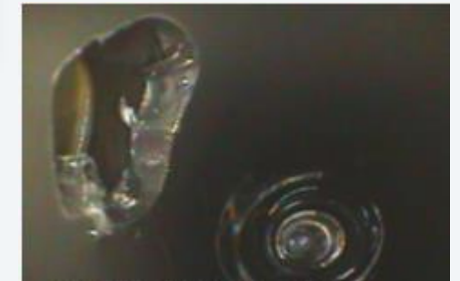
Service connection with illegal connection
